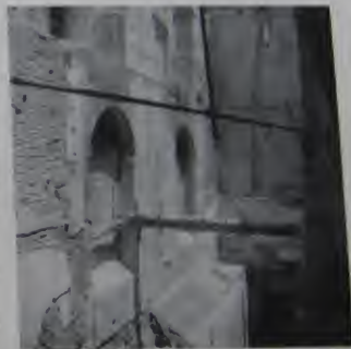
Fig. 38. Interior of the church, showing the structure of the apse.
